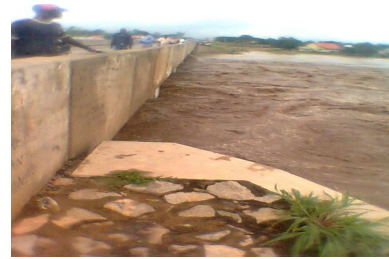
Plate 2. The 2011 Flood water under Nukkai bridge along Jalingo-Wukari road
