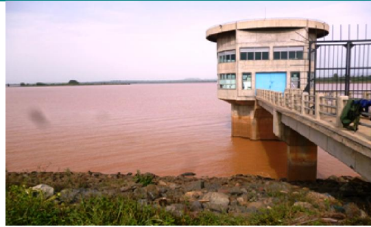
Fig 5: Part of Koga Dam Water Body and Dam Intake Tower
