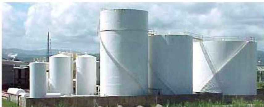
Figure 1.5. Cylindrical tanks in Yabucoa, Puerto Rico.
