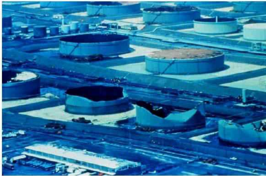
Figure 1.6. Collapsed tanks in St. Croix after hurricane Hugo (1989).
