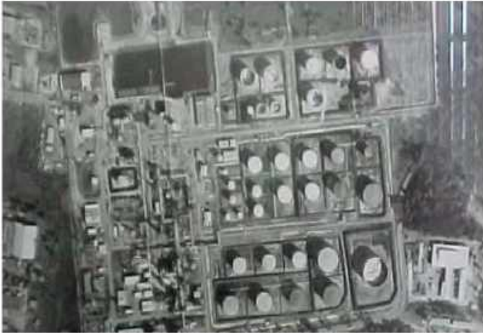
Figure 1.1. Aerial view of a tank farm located in Puerto Rico (Caribbean Petroleum).
