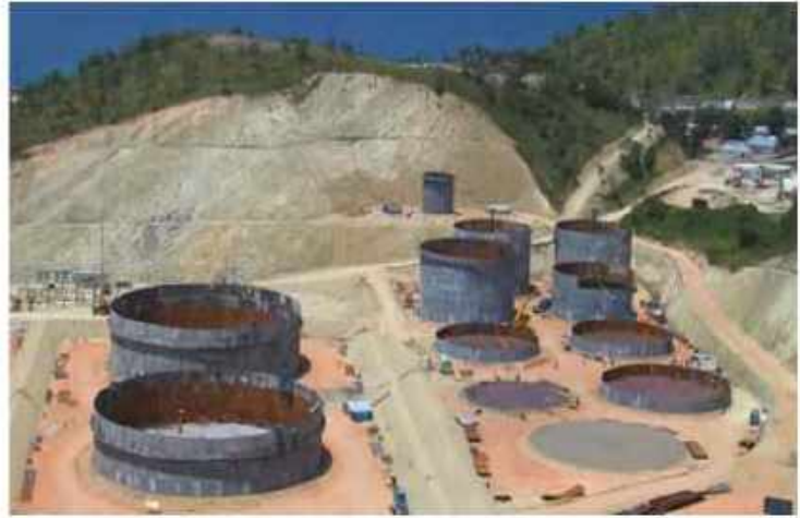
Figure 1.2. Tank farm located in Saint Lucia, during construction.
