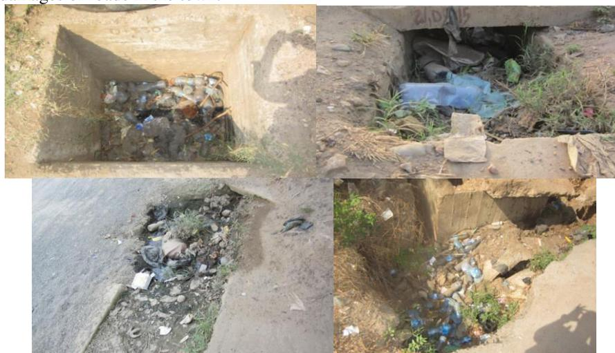
**Pic 1.** The blocked storm drainages system by wastes and damaged roads in Gambella town.
