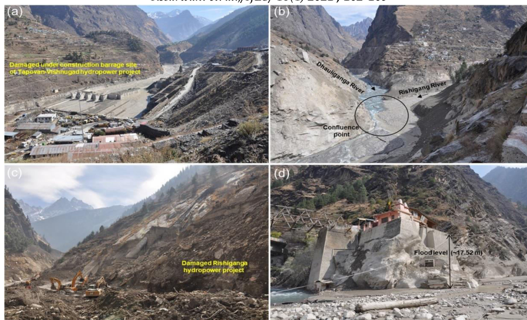
Fig 2. (a) Damaged under construction barrage site of Tapovan-Vishnugad hydropower project at Tapovan village (520 MW, owned & operated by National Thermal Power Corporation Limited-NTPCL), (b) confluence zone of Dhauliganga and Rishiganga rivers at Raini village (c) Rishiganga hydropower project (13.2 MW, owned & operated by Kundan Group, New Delhi) at Raini village, and (d) flood level during the disaster at Vishnu Prayag site (1458 m a.s.l.).
