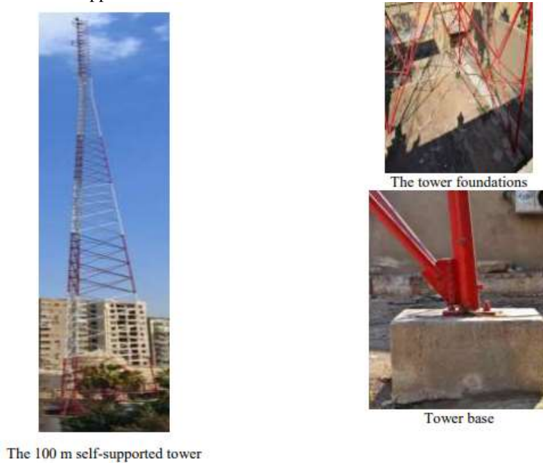
Fig (1): The components of self-supported tower
